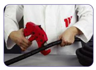
2 Cut the end of the hose in a perpendicular direction, using the manual cutter.
